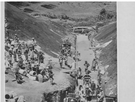
Railway construction workers building a culvert at Mile 398, Kikuyu Source: Nairobi National Museum
