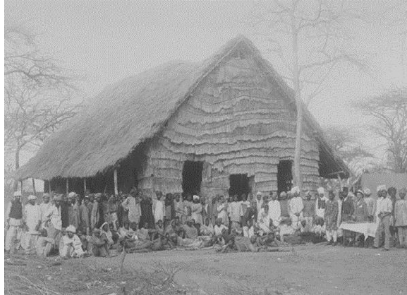
A Church in Kibwezi that served as a hospital for Railway construction labourers Source: Nairobi National Museum
