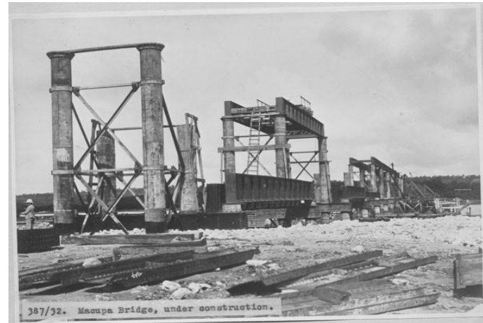
Construction workers on site
