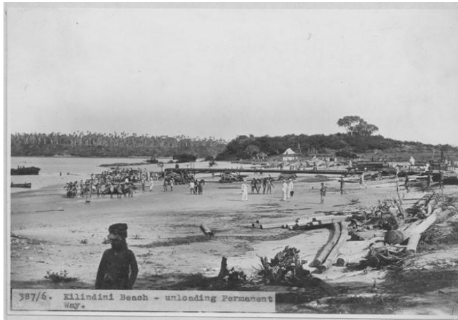
Unloading of construction materials at Kilindini port, Mombasa
